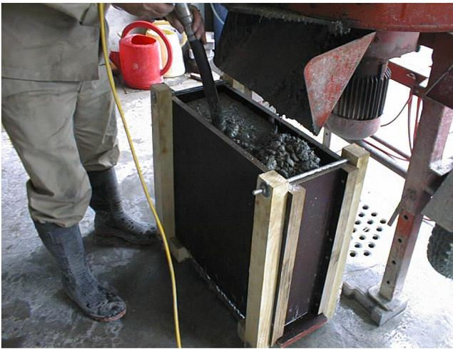
*Fig. 1 Fabrication of a wall element*
